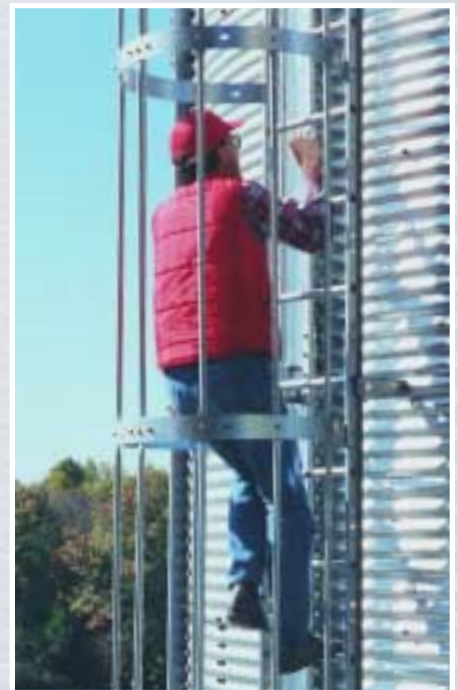
Ladder Safety Cage is standard for ladders on bins with an eave height of over 20 feet (6.1 meters).
